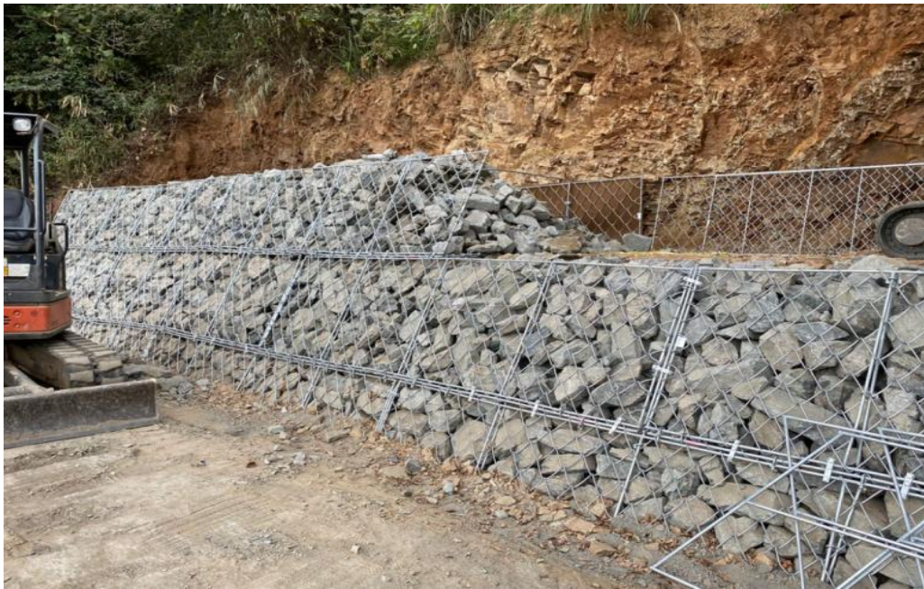
Figure 6.11 Gabion Check Dam (Source: Pinterest Gabion Check Dam)
