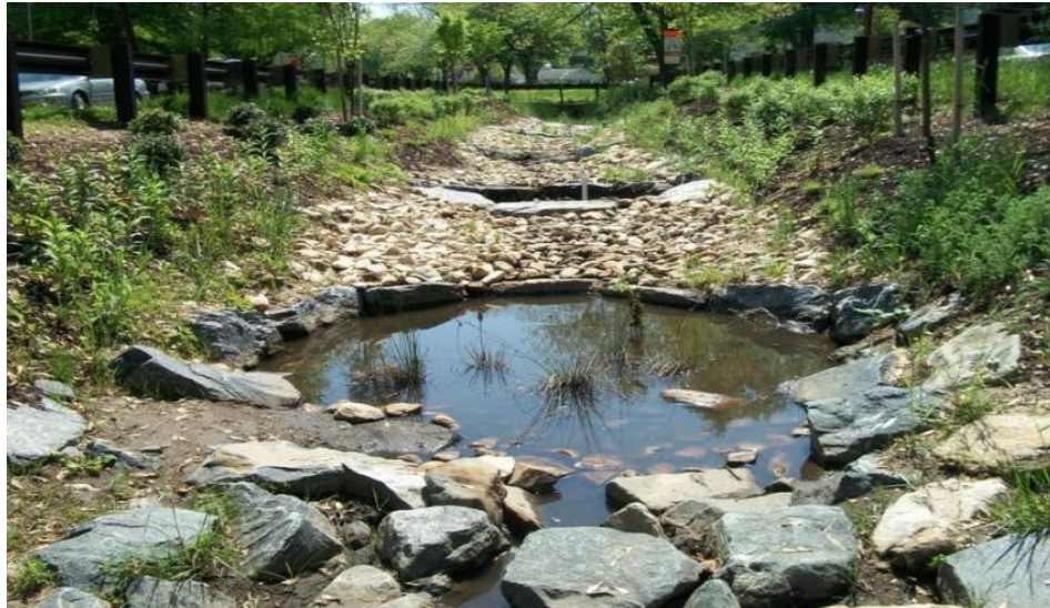
Figure 6.10 Loose Stone Check Dam (Source: Flickr Loose Stone Check Dam)
